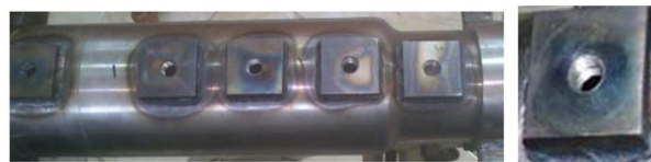
Fig. 3 Pieces of reinforcement
