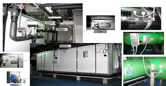
Fig. 2 AHU of clean room
