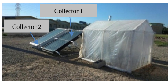
Fig. 2 Real view of greenhouse and heating system
