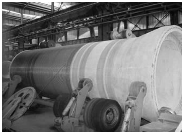
Fig. 5 Pre-stressing of concrete pipe with spiral rebar
