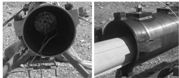
Fig. 9 Installation and placement of fuel
