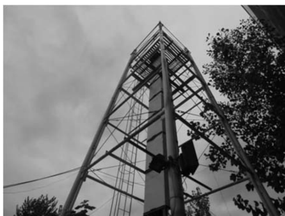
Fig. 2 A total view of the drop hammer apparatus
