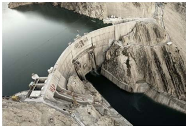
Fig 4 Karun 3 dam and its reservoir and appurtenant
